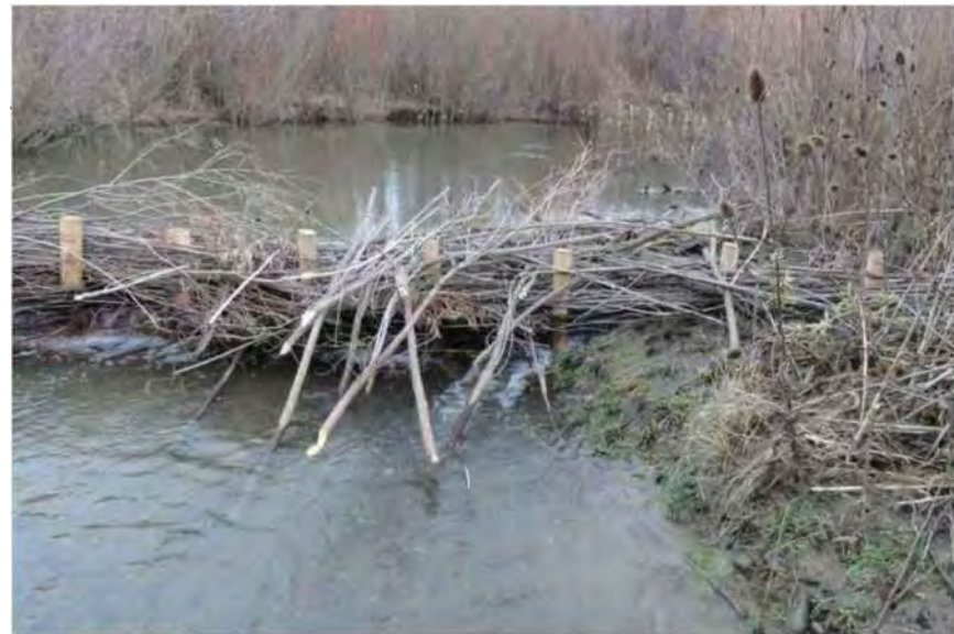
EXAMPLE BDA POST LINE WITH WILLOW WEAVE, NOAA FISHERIES, "WORKING WITH BEAVERS TO RESTORE SALMON HABITAT", 2003
