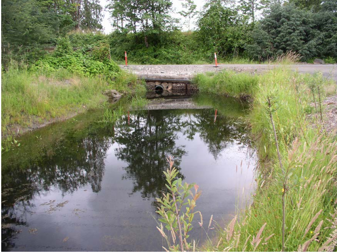
Figure 1. View looking west of existing crossing.
