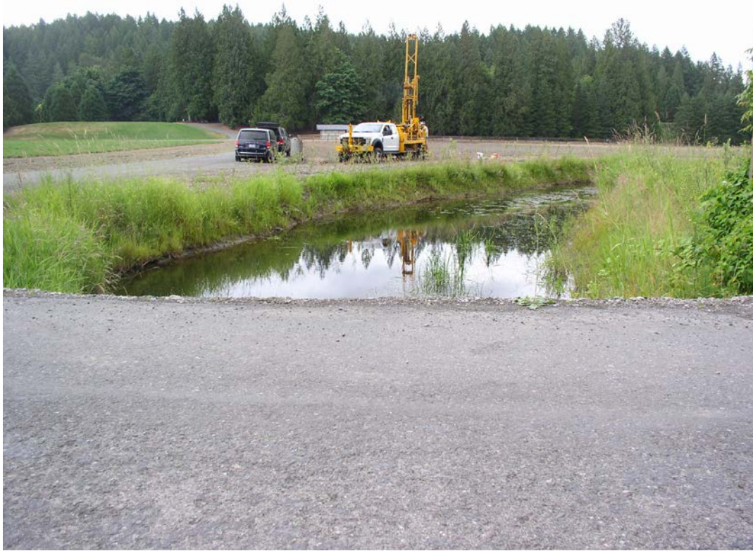
Figure 3. View looking east of drill rig set up at DH1.
