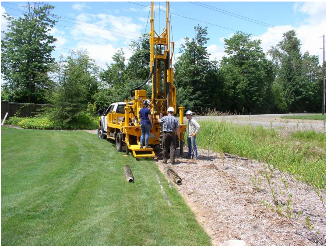
Figure 4. View looking northwest of drill rig set up at DH2.
