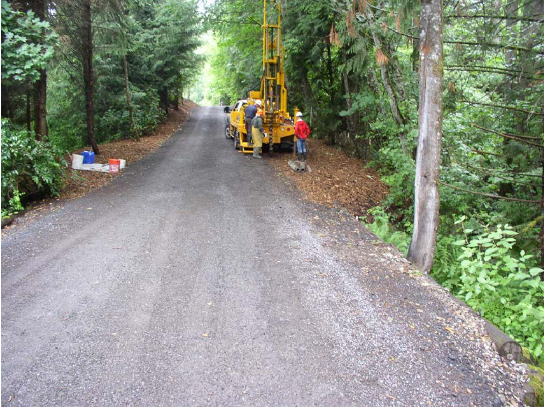
Figure 3. View looking north of drill rig set up at DH1.
