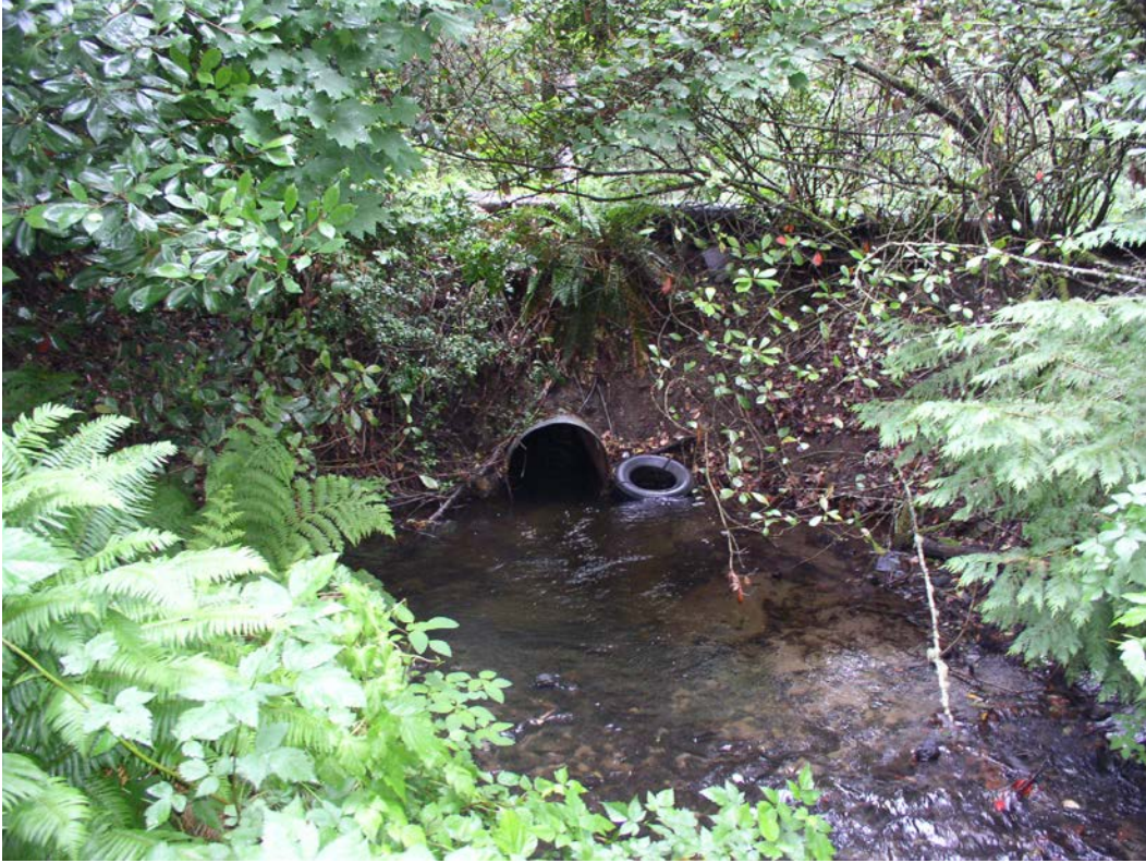
Figure 1. View looking east of existing crossing.
